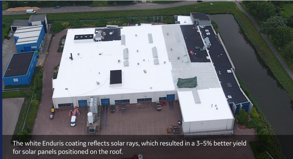
The white Enduris coating reflects solar rays, which resulted in a 3–5% better yield for solar panels positioned on the roof.
